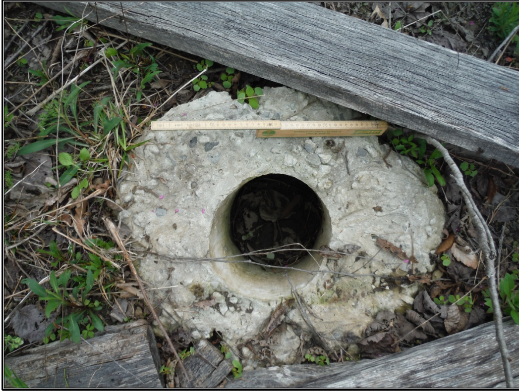
Figure 12. Example of a poured concrete support for wood post foundation piers.
